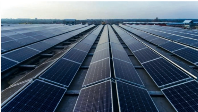
Using of solar power during the day to run Hybrid lehr
